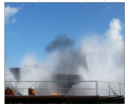
Deck Integrated Fire Fighting DIFF
