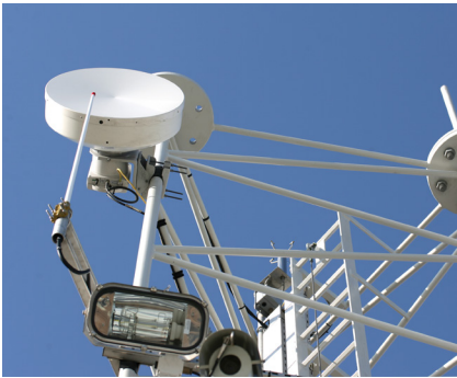
Microwave Radio Link system
